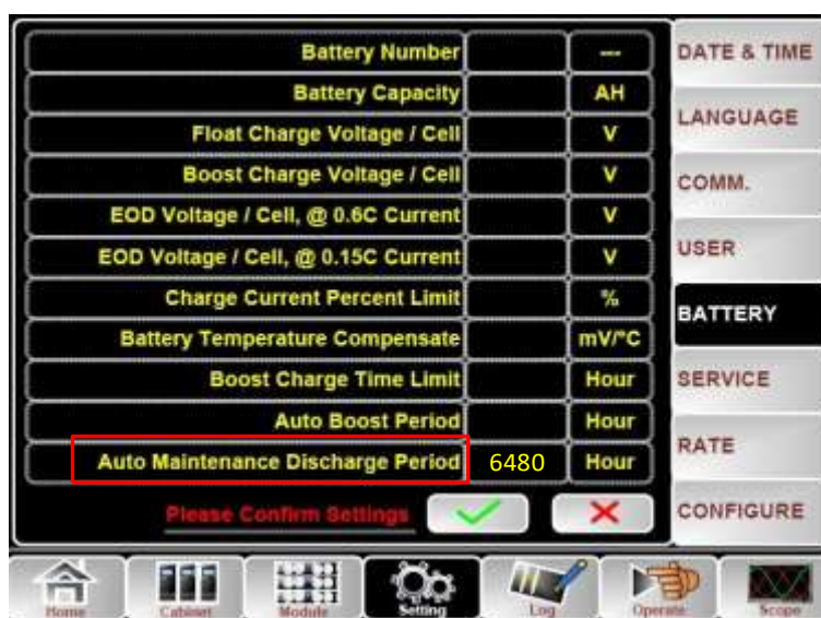
Figure4-4 Setting period for battery auto discharge
